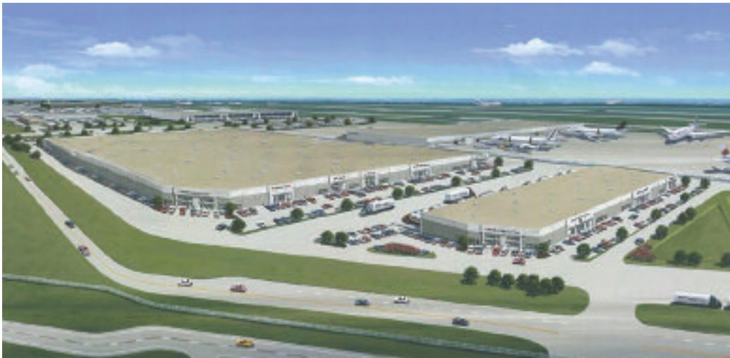
KCI Intermodal Business Centre
